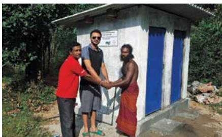
Rathugala Water & Sanitation Project
