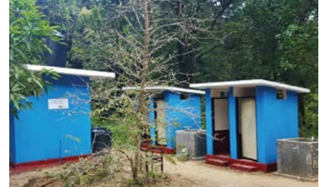
Water & Sanitation Project - Rathugala
