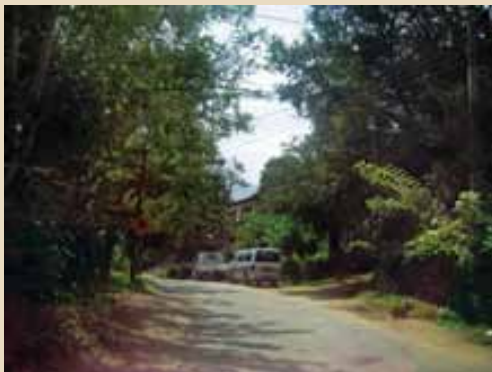
The image shows the current status of the road before the commencement of rehabilitation and improvement
