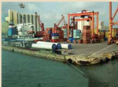
The image shows the damaged section of the UCT
