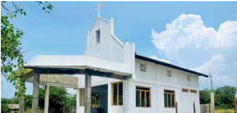
St. Anthony's Church, roof construction in Mannar
