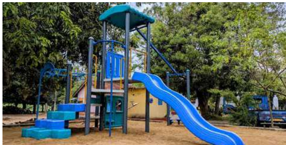
Construction of a safe and durable playground base at Kirimatiyawa Junior School
