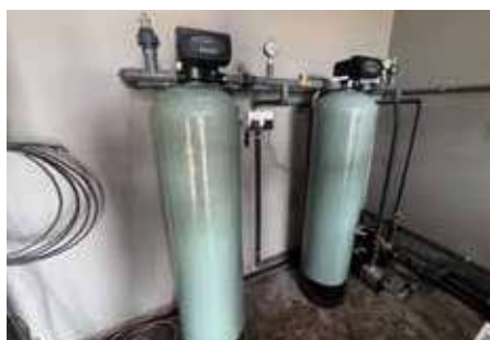
Reverse Osmosis (RO) Water Purification at Kebitigollewa Solar Power Plant
