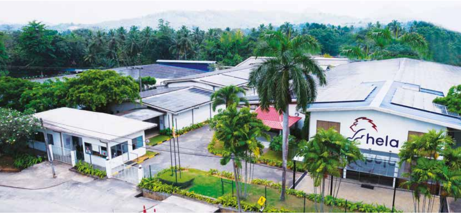
Hela Mawathagama manufacturing facility
