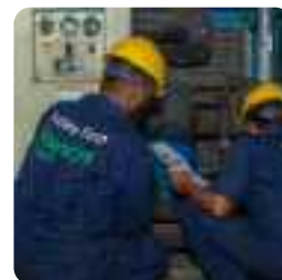
Routine maintenance checks on plant and equipment
