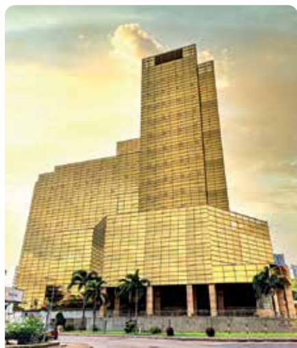
Sampath Centre building after renovation
