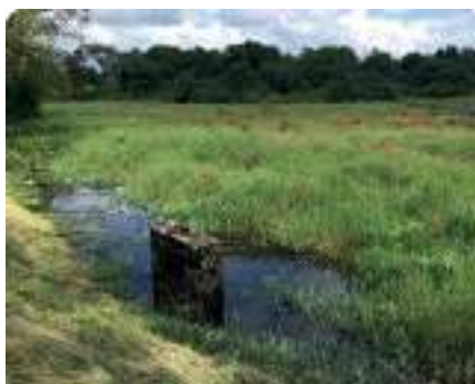
Pre-condition of the tank
