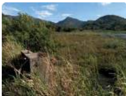
Pre-condition of the tank
