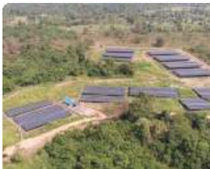
Ground mounted solar power project at Maho. Project capacity: 3 MW
