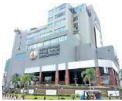
Before refurbishing the Bank's Head Office
