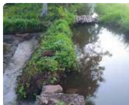
Pre-condition of the canal system
