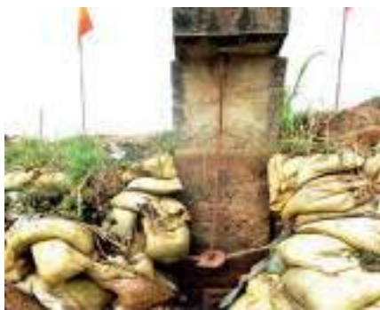
Pre-condition of the tank bund and sluice
