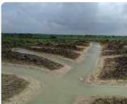
Newly developed canal system in the project site
