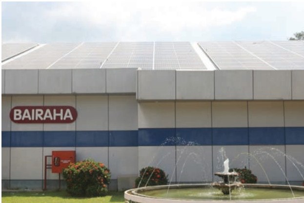
Solar panels installed at the rooftop of the Processing Factory
