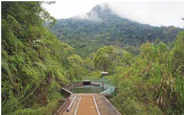
Closed head race channel and protective hand rails
