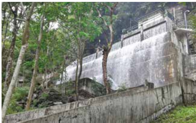
Concrete channel for Forebay spill way to prevent soil erosion
