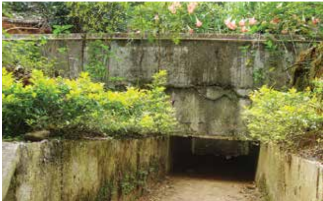
Drainage system constructed under the channel
