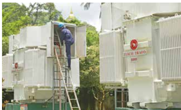
Regular maintenance work of Transformers
