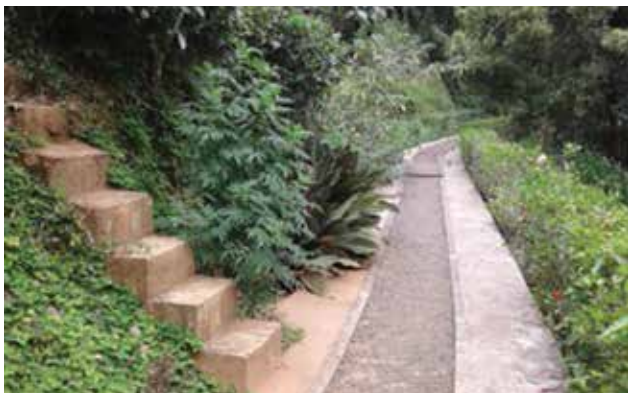
Concrete steps to facilitate movement of inhabitants across the channel
