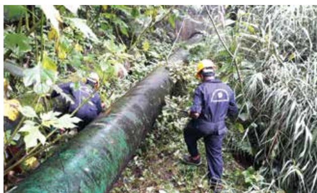
Regular Inspection of Penstock line
