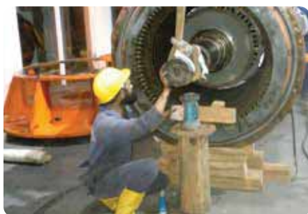
Break-down repair at Kiriwaneliya MHP
