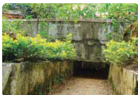
Drainage system constructed under the channel
