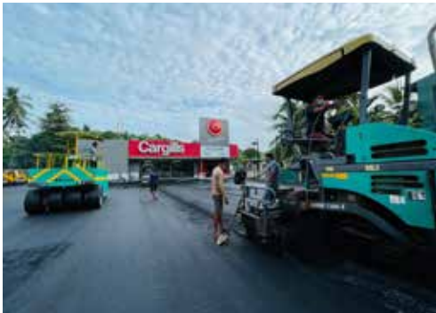
First ever car park in Sri Lanka built with Plastic Modified Asphalt Concrete (PMAC) in Walgama, Southern Sri Lanka
