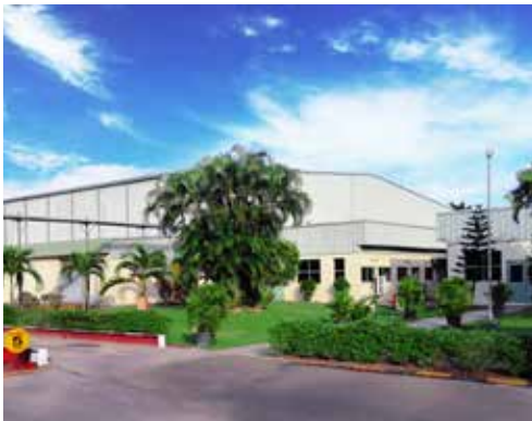
KIST processing facility in Katana
