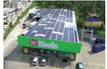
Solar power converted Keells outlet
