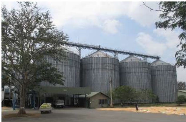
Storage Silos and Drying Plant for Paddy and Maize
