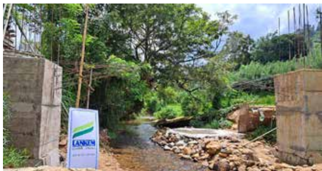
Restoration of Bridge in Varaniyawatta village
