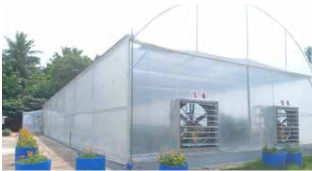
Fully automated Poly tunnel at Pannala
