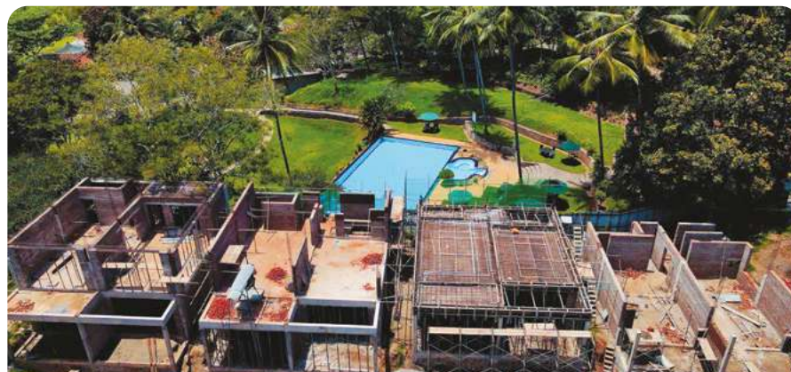
Ongoing construction of villas at RHL.
