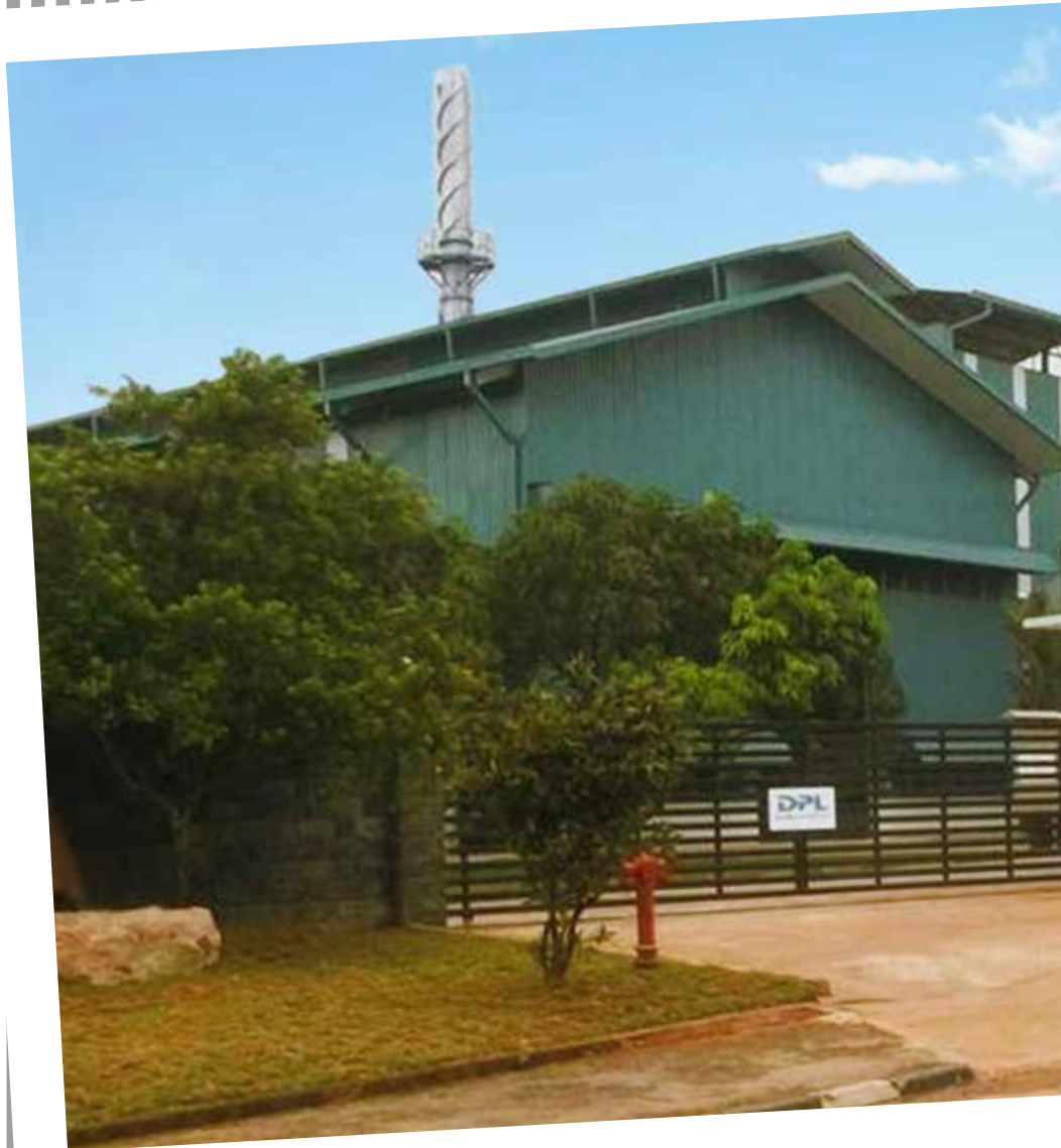
D P L Premier Glove Factory at Biyagama
