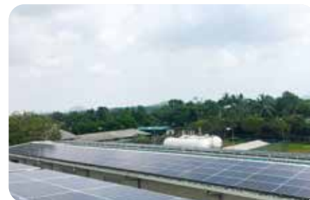
Solar PV systems successfully installed in all factory roofs
