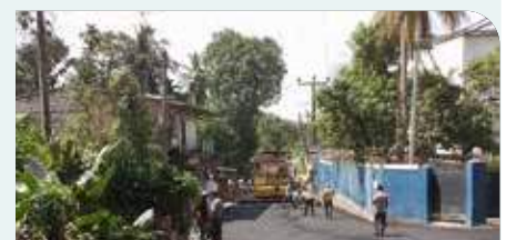
Reconstruction of the adjoining road of Eheliyagoda Factory
