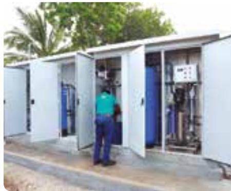
*The customised PureHydro® water purification solutions with Reverse Osmosis Technology, comes with an output capacity of 5000 litres a day.*
