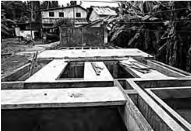
Construction of Effluent Treatment in progress at Frosceter Estate, Govinna
