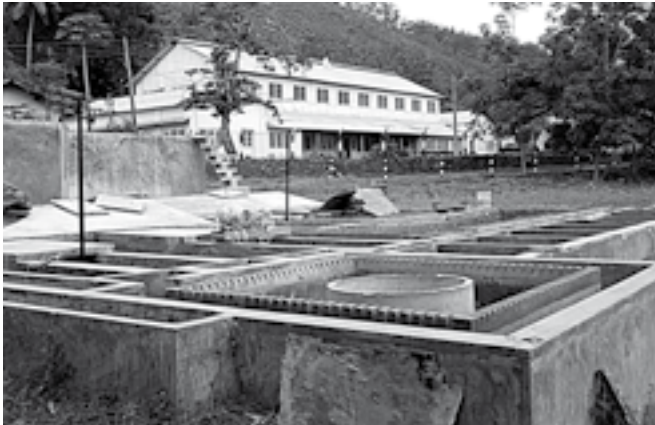
Effluent Treatment Plant at Kobowella Estate Rubber Factory, Govinna
