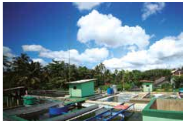
Effluent Treatment Plant - Centrifuged Latex Project - Udapola Estate
