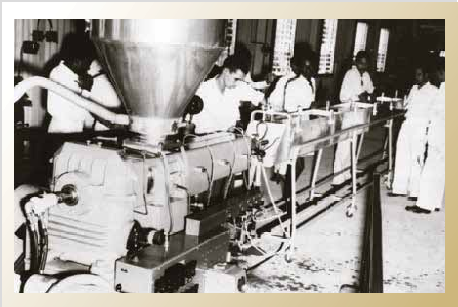
Machinery inspection by Browns Group Engineering Department.
