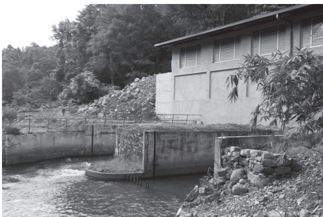
2.0 Mw Giddawa Hydro Power Plant in Digana
