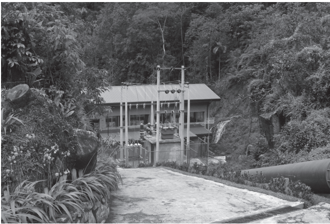
2.4 MW Magalganga Hydro Power Plant in Maliboda
