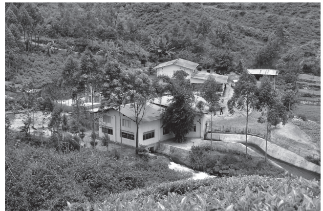
2.6 Mw Agraoya Hydro Power Plant in Lindula
